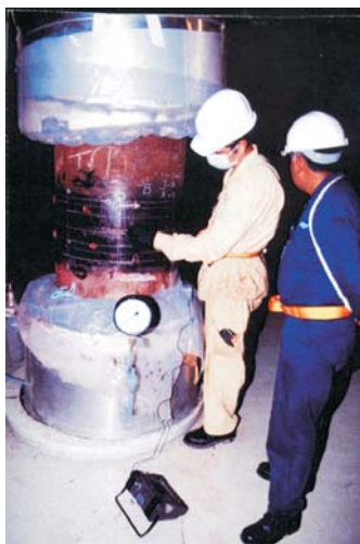
Ultrasonic inspection of welds of a piping system
