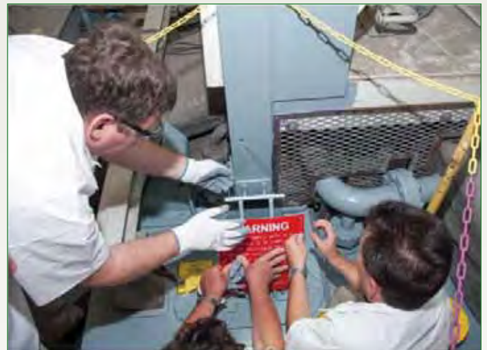
During a July 2012 PPRA monitoring visit to the Savannah River Site's K Reactor, U.S. experts installed the first PPRA seal at a shutdown U.S. reactor in over a decade.
