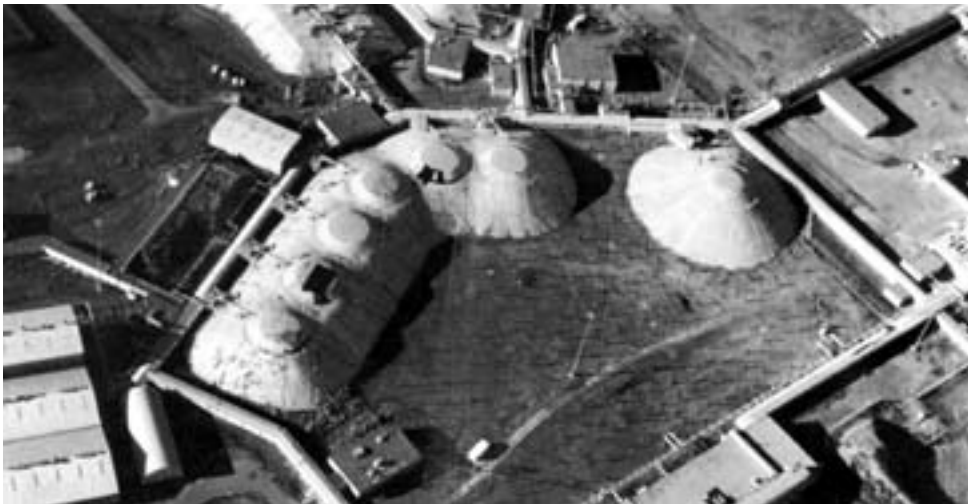
Figure 5.3. Warhead dismantlement cells, Pantex plant, Amarillo, Texas. 265 The circular concrete structures, "gravel gerties," cover cells where warhead components containing conventional high explosives are assembled and disassembled. Pantex
